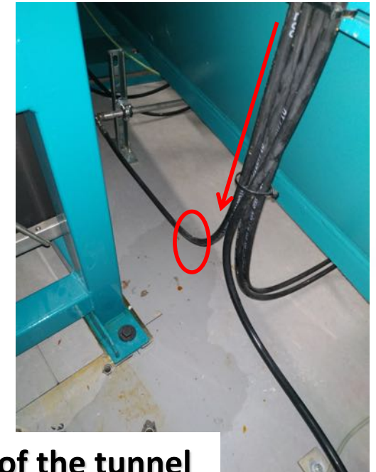
Exuding water along the hose (1 drop/sec)
