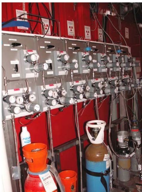
Figure III.20. The array of gas bottles outside the experiment hutches
