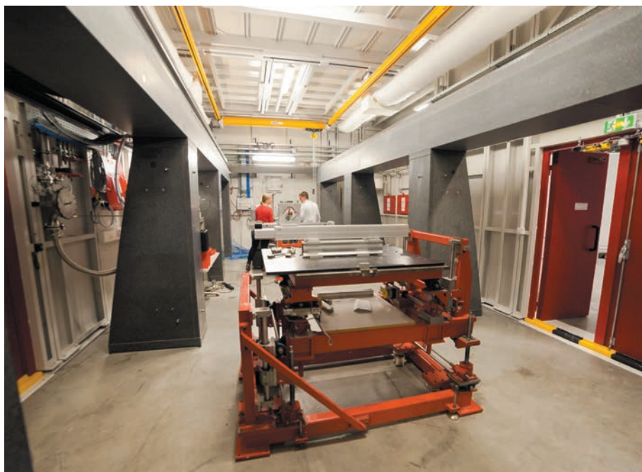
Fig. 2: ID31 experimental hutch during construction of the beamline.
